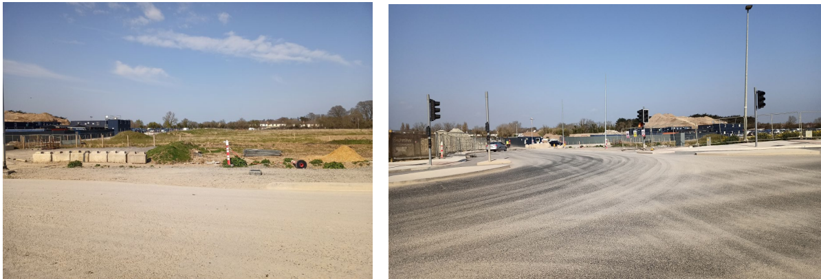
Figure 14.23: Views of surrounding established housing in the background (a) Priory Wood against the site's northern boundary and (b) The Links to the west of site as visible from the DRR. Ongoing Development works dominate the foreground.
